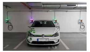
on Foxtrot system - which may be in another building or even in another city. This creates a network of charging stations that are automatically regulated and controlled. This approach allows the operator to avoid power outages or even penalties issued the power distributor while making sure that the customer benefits from automatic energy cost savings, and has a complex overview of all charging stations while being able to control, manage and verify the relevant charging accesses.
