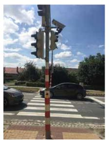
errors. The red light passing monitoring system RedCon also provides data such as the number of vehicles, photos and recognized vehicle license plates. The iSmartCity.cz system may also be used to control individual streetlamps or group of lamps and to group them into various time scenarios, etc. Other devices may be connected as well providing that these are equipped for such connection and may be safely operated under this regime.
