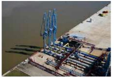
Special oil feeders must balance the filling level of the tanker as it can drop down up to 18m. The capacity of the anchoring area where the fuelling takes place is 8,000 - 12,000 m² / hour.
