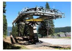
pod Šněžkou in the Krkonoše mountains in the ski resort Zahrádky (Gardens) where a cable car line manufactured by Leitner was installed. This cable car was previously used in the Alps in Obertauern. It is a four-seater cable car with cabins which hang on a fast moving rope. When passengers need to get in or out, the cabin is removed from the fast rope and hung on a slow rope to allow comfortable boarding and exit.
